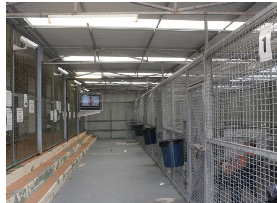
Long Bay holding yard
